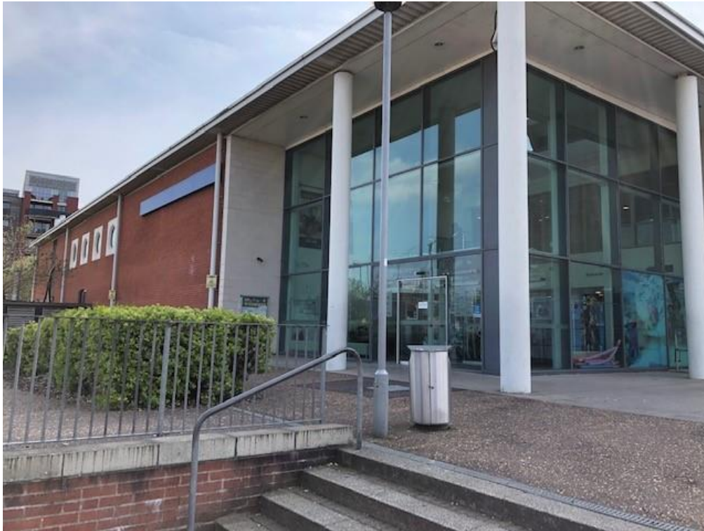
Front door access to the site building.
