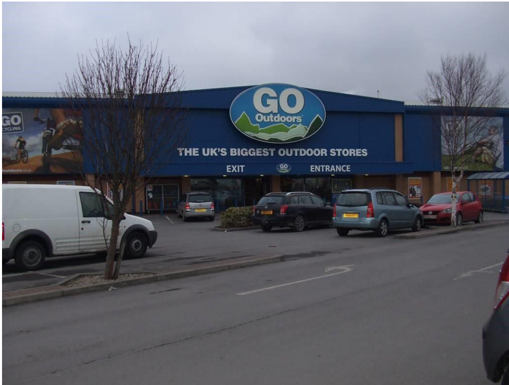
Front doors to the site building.
